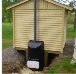
Note that the tank is not strong enough to support the toilet. The toilet needs to be supported by the floor or bench.
